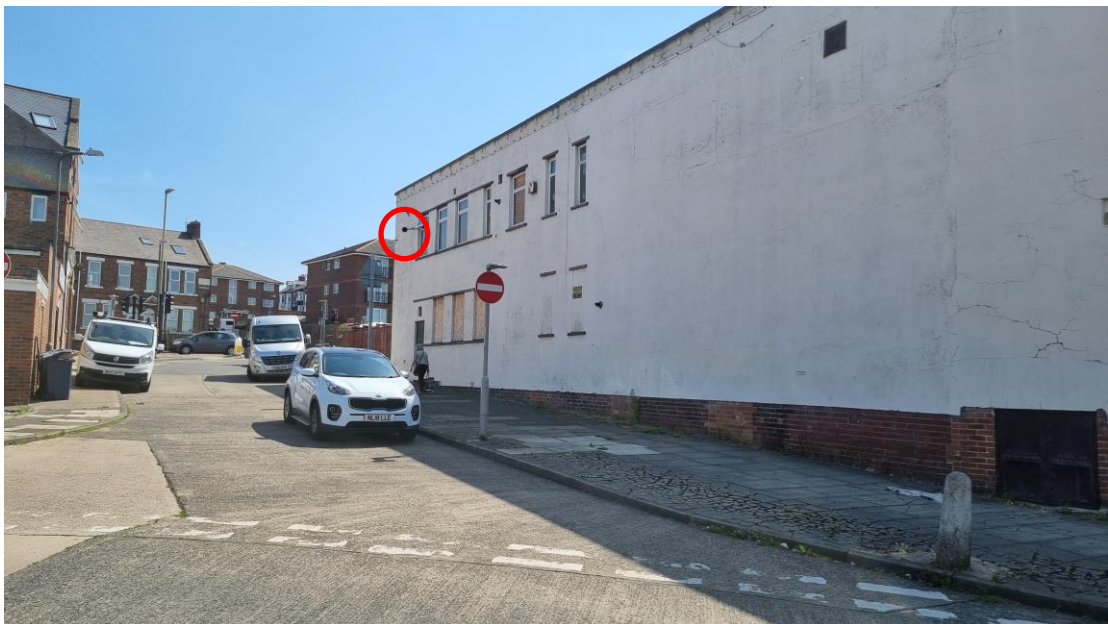
Photograph 3: Microphone position - 1 st floor on northern elevation
